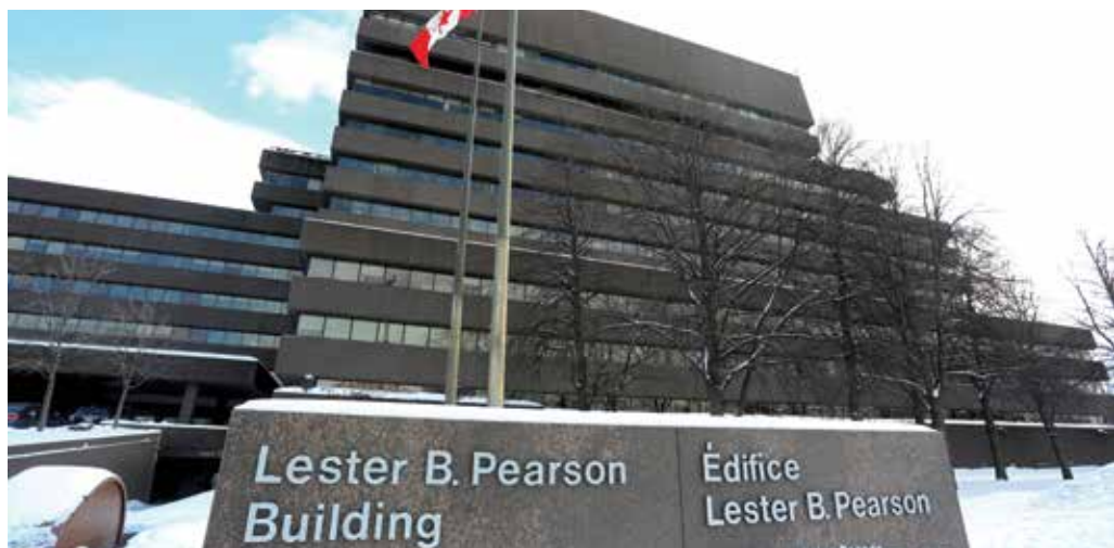
Global Affairs Canada, headquartered in Ottawa's Pearson Building, has missions in Japan, Mexico, and Senegal, among others, that are rated in 'critical' condition. The Hill Times photograph by Andrew Meade
