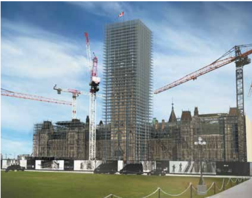
An artist’s rendering of the scaffolding that will cover Centre Block’s southern façade—sans the trompe l’oeil tarping that’s to come—and the steel frame that will surround the Peace Tower by late 2026 or early 2027. Image courtesy of Public Services and Procurement Canada
