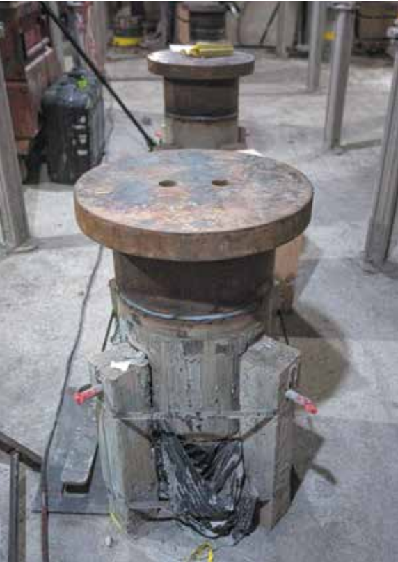
Two steel piles, which have been drilled and capped off, on the sub-basement level. They are two of a cluster of four which will serve as one of many points onto which the building load will be transferred ahead of excavations underneath Centre Block.
