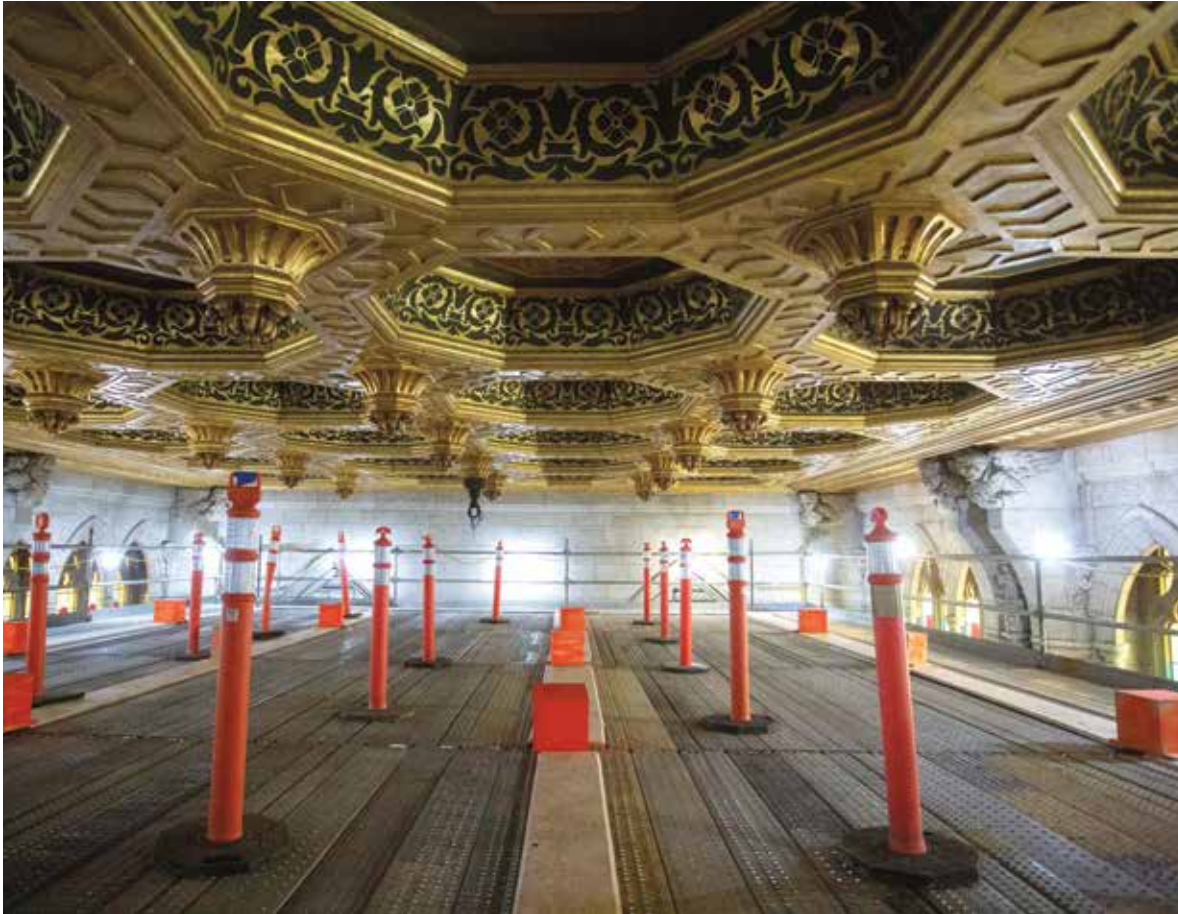
Inside the belly of the Senate: the Red Chamber is going through major restoration work. Construction workers were surprised to find that the foundation was made of rubble. Work is underway to reinforce its foundation with cement. The Hill Times photograph by Andrew Meade
