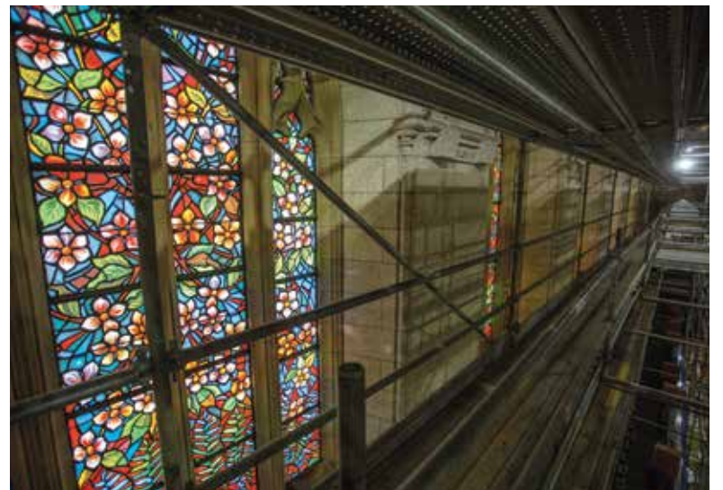
Centre Block is now overrun with scaffolding, but the stained-glass windows that are a feature of the House of Commons Chamber haven't completely been obscured. The Hill Times photograph by Andrew Meade
