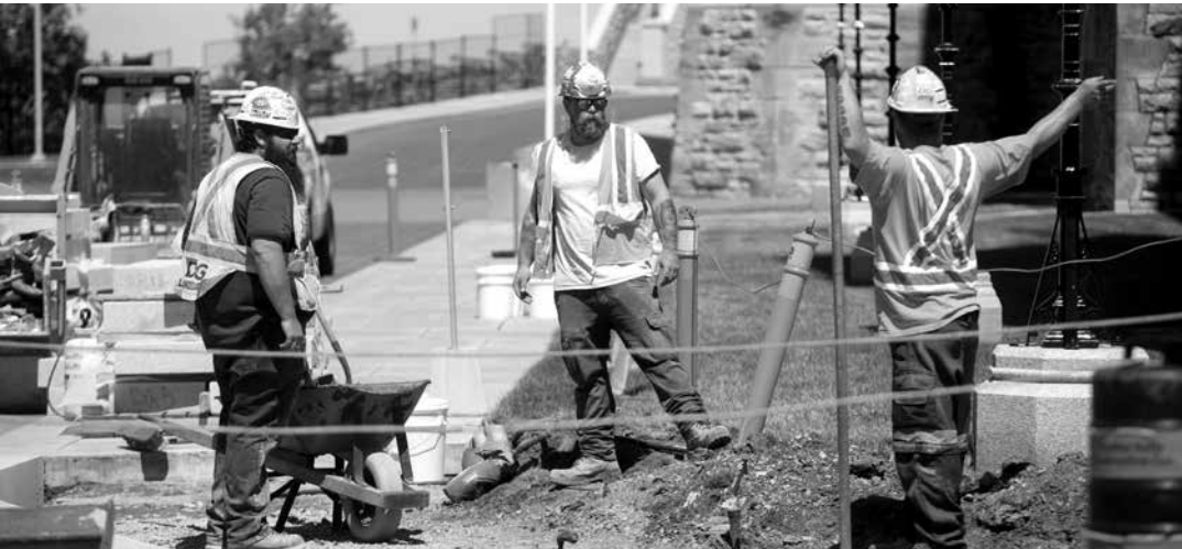
Construction workers shoot the breeze while working on Parliament Hill.
