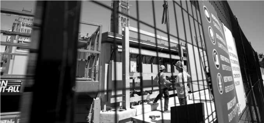
Hill construction workers pictured working on the Hill.
