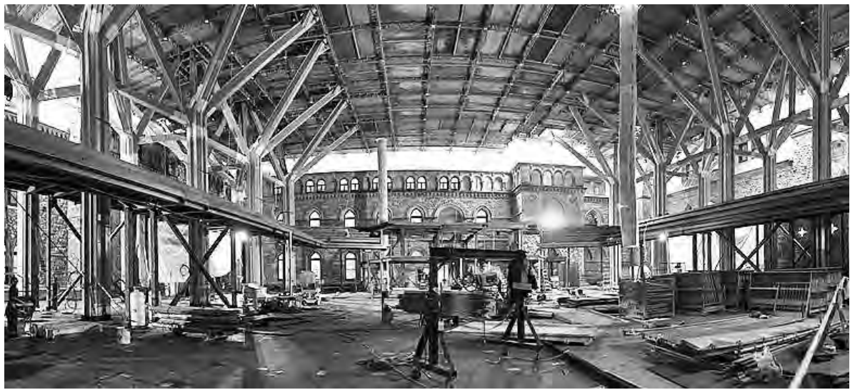
New House Chamber Coming: The completed steel framing for the interim House of Commons Chamber, including the viewing galleries, is pictured in the West Block's courtyard on March 31. Concrete is currently being poured and installation of the glass-domed roof is ongoing, with protection put up (as shown) to allow work on the interim Chamber to continue at the same time. Photograph courtesy of Public Services and Procurement Canada
